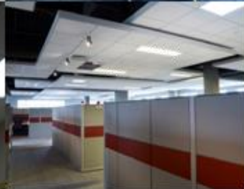
Optima Engineering MEP Firm Charlotte, NC
