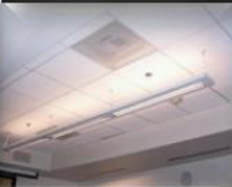
Southern Cal Edison Utility Services Office Irwindale , CA
