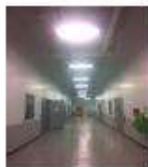
24v DC HIGH BAY ALUMALIGHT 6 LAMP T8 FLUORESCENT LAB LIGHTING (NEW FIXTURES TO REPLACE EXISTING HID)
