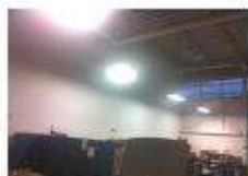
24v DC HIGH BAY ALUMALIGHT 6 LAMP T8 FLUORESCENT LAB LIGHTING (NEW FIXTURES TO REPLACE EXISTING HID)
