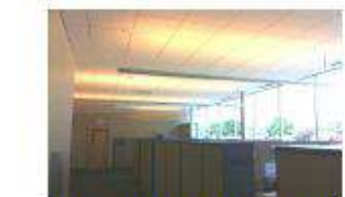
24v DC OFFICE AREA LIGHTING (RETROFIT OF EXISTING TS LAMP FIXTURES)
