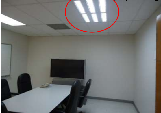
2x4 60W Troffer (replacing 160W)
