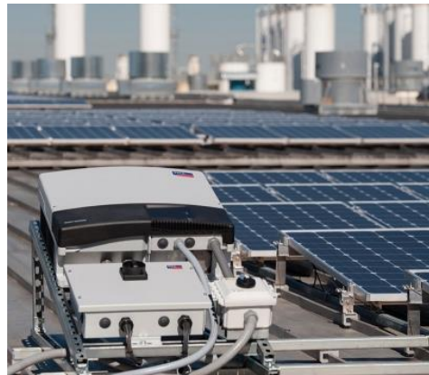
Roof-mounted inverters
