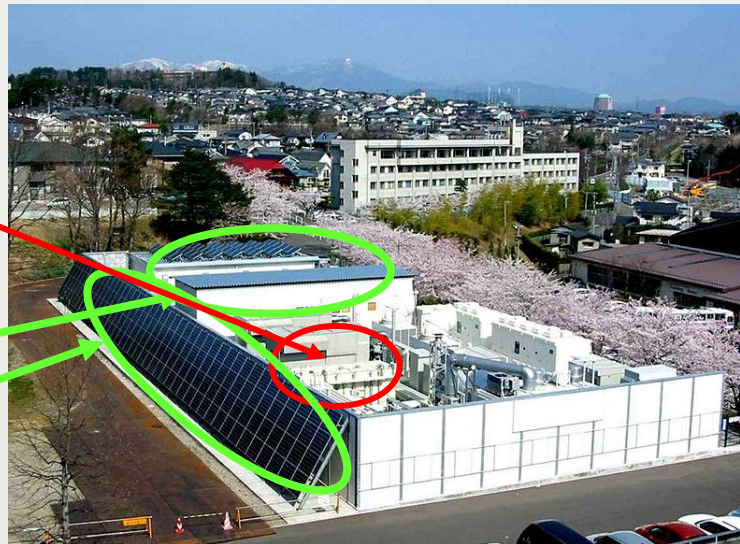
Microgrid in Sendai
