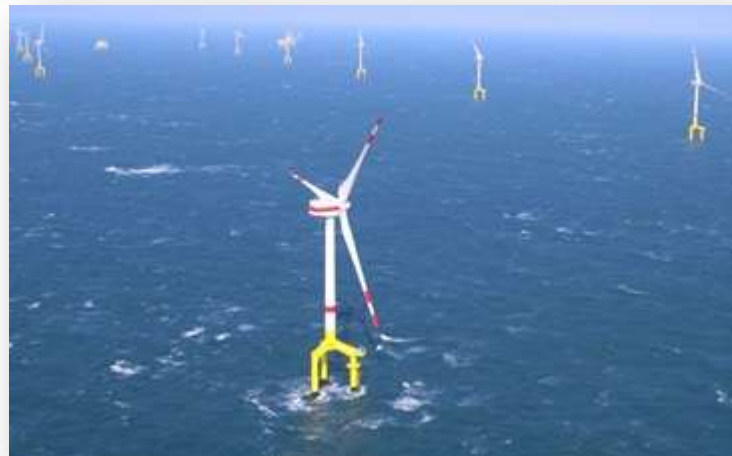
BARD Offshore 1: 80 turbines 400 MW (2013)
