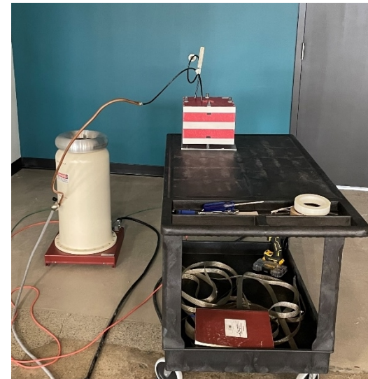
In-house MV Hipot testing
